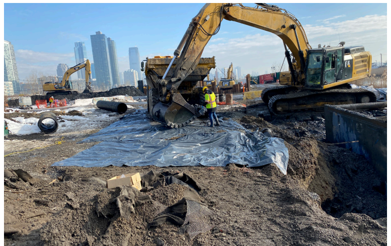
Soil Remediation and Dewatering
